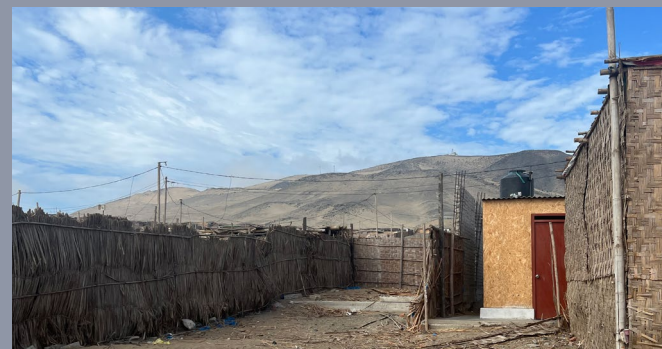
Back of Learning & Soup Kitchen Future Daycare Site
